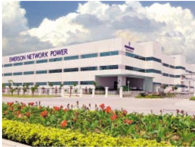
Emerson Network Power, Shenzhen. Courtesy of Emerson.
